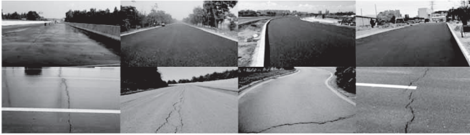
Figure 3 Photos taken at the construction site.
